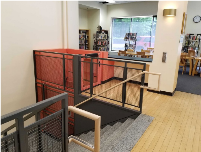
View of the newly installed lift at the Philadelphia City Institute Library.
