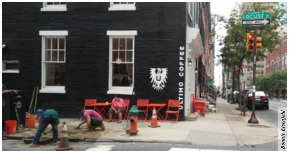
Workers repair the unpaved section of sidewalk in front of the Ultimo Coffee Bar.
