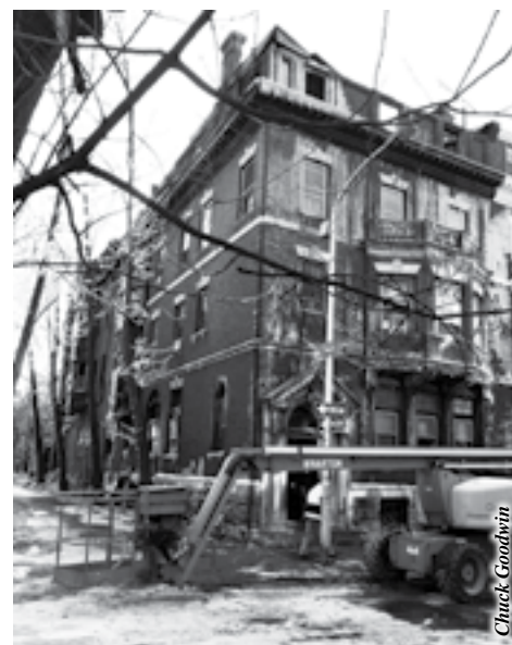
Devastation in the aftermath of the fire.
