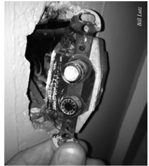
Old push button light switches are indicators of old knob and tube wiring.
