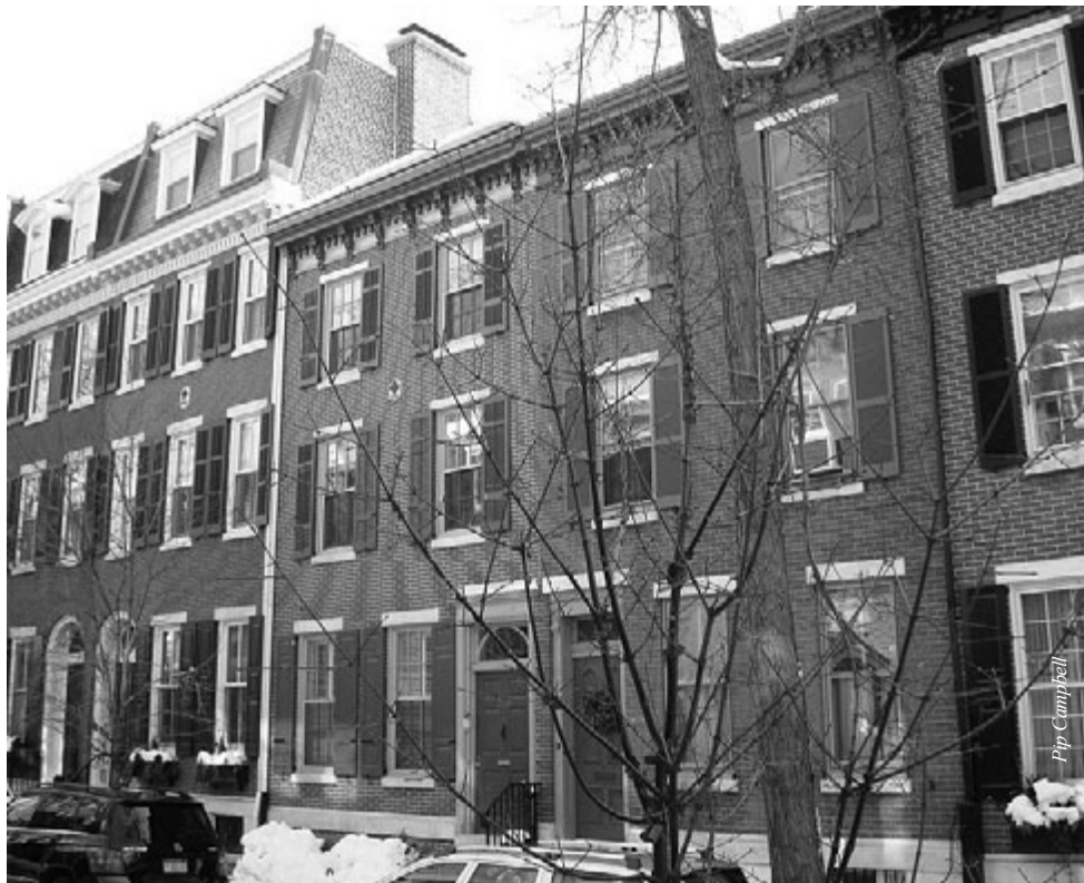
Most of the houses on the 2100 block of Delancey Place were built in the 1840s-1850s by local bricklayers on speculation. As neighborhoods expanded east from the Schuylkill River, the houses on this block of Delancey were built as residences for the middle class.
