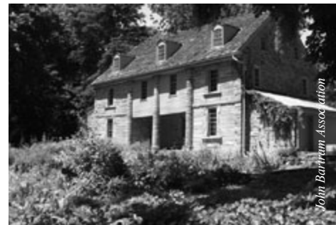
John Bartram designed and built this house over nearly 50 years (1728 to 1777) out of local river stone.
