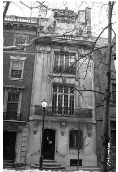
Horace Trumbauer designed 1629 Locust Street for Edward Collings Knight, Jr., a prominent socialite and the son of Edward C. Knight, Sr., a wealthy sugar refiner. Built in 1902, the limestone façade of this Beaux Arts mansion is unusual for the Rittenhouse Square neighborhood.
