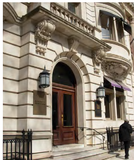
Barney's at 10 Rittenhouse: Built in 1901 in the Beaux Arts style, James Harper's mansion – whose facade has been preserved – later became the Rittenhouse Club.
