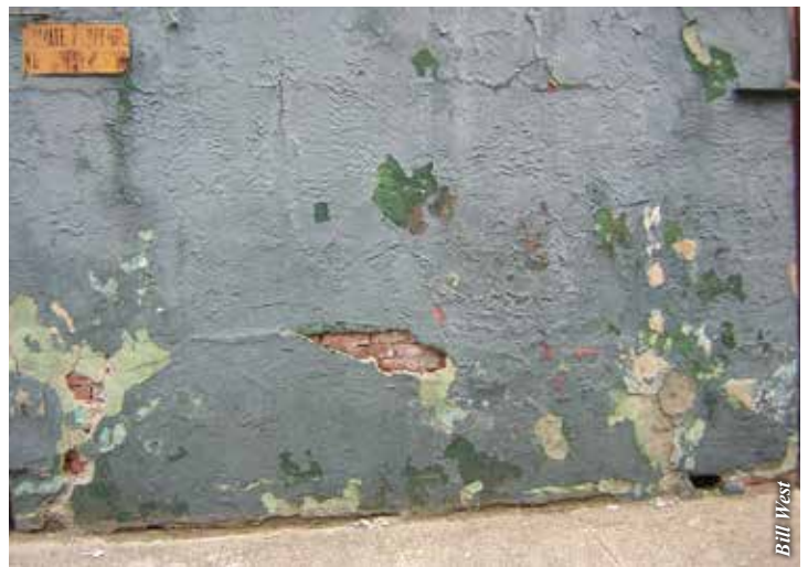
1700 block of Delancey. This wall no longer looks like this.
