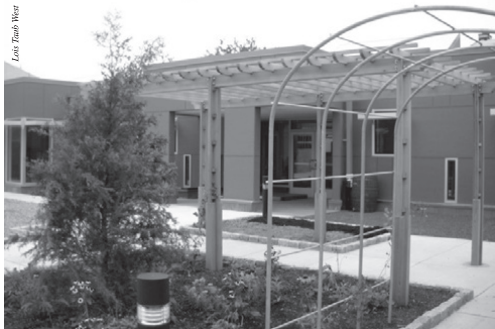
There will be a ribbon-cutting at the Philadelphia School's new Ellen Schwartz & Jeremy Siegel Early Childhood Education Center at 25 th and South streets on September 21.
