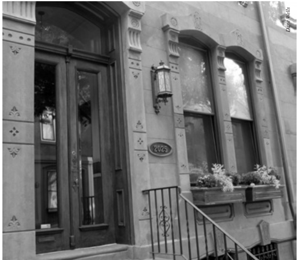
The work done to restore and maintain this property showed the owner's care. The door was recently refinished; the window boxes are a nice touch; and the stucco is in excellent condition.
