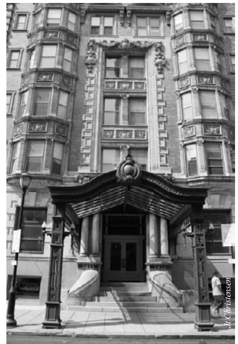
The beautifully restored façade of The Belgravia on the 1900 block of Chestnut Street was designed by Frederick Webber and built in 1902.
