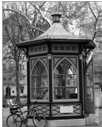
The Park Guard kiosk was saved from demolition, restored and installed in Rittenhouse Square.
