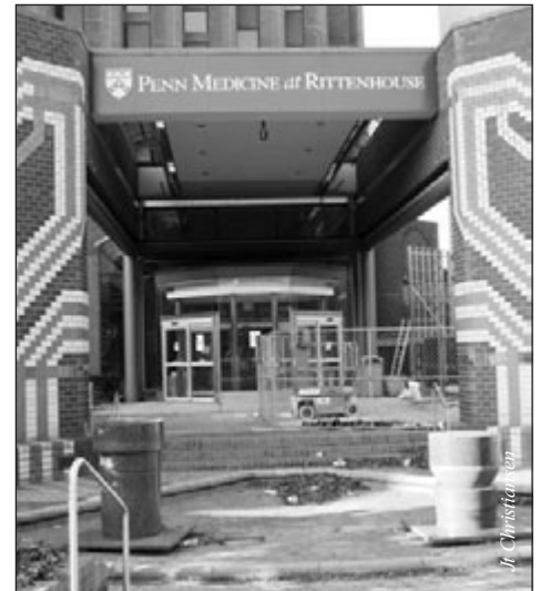
Under construction is the new entrance to Penn Medicine at Rittenhouse.
