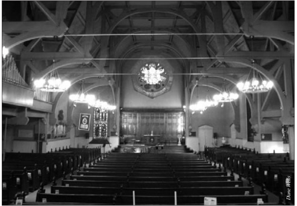
The sanctuary of the First Unitarian Church features hammerbeam trusses.
