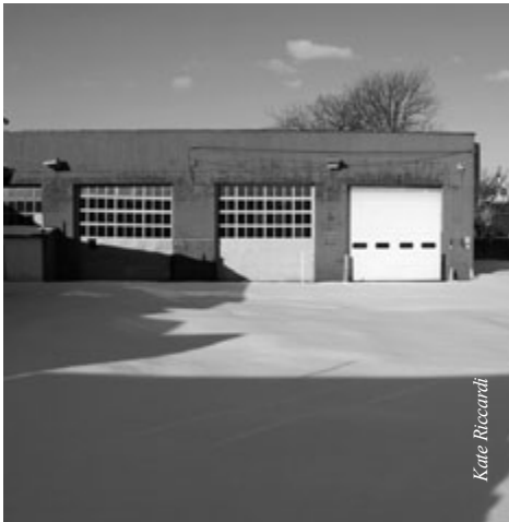
The current view of the existing four-bay industrial garage at 2501 South Street that will be recycled into a new flexible Multipurpose Space for The Philadelphia School.
