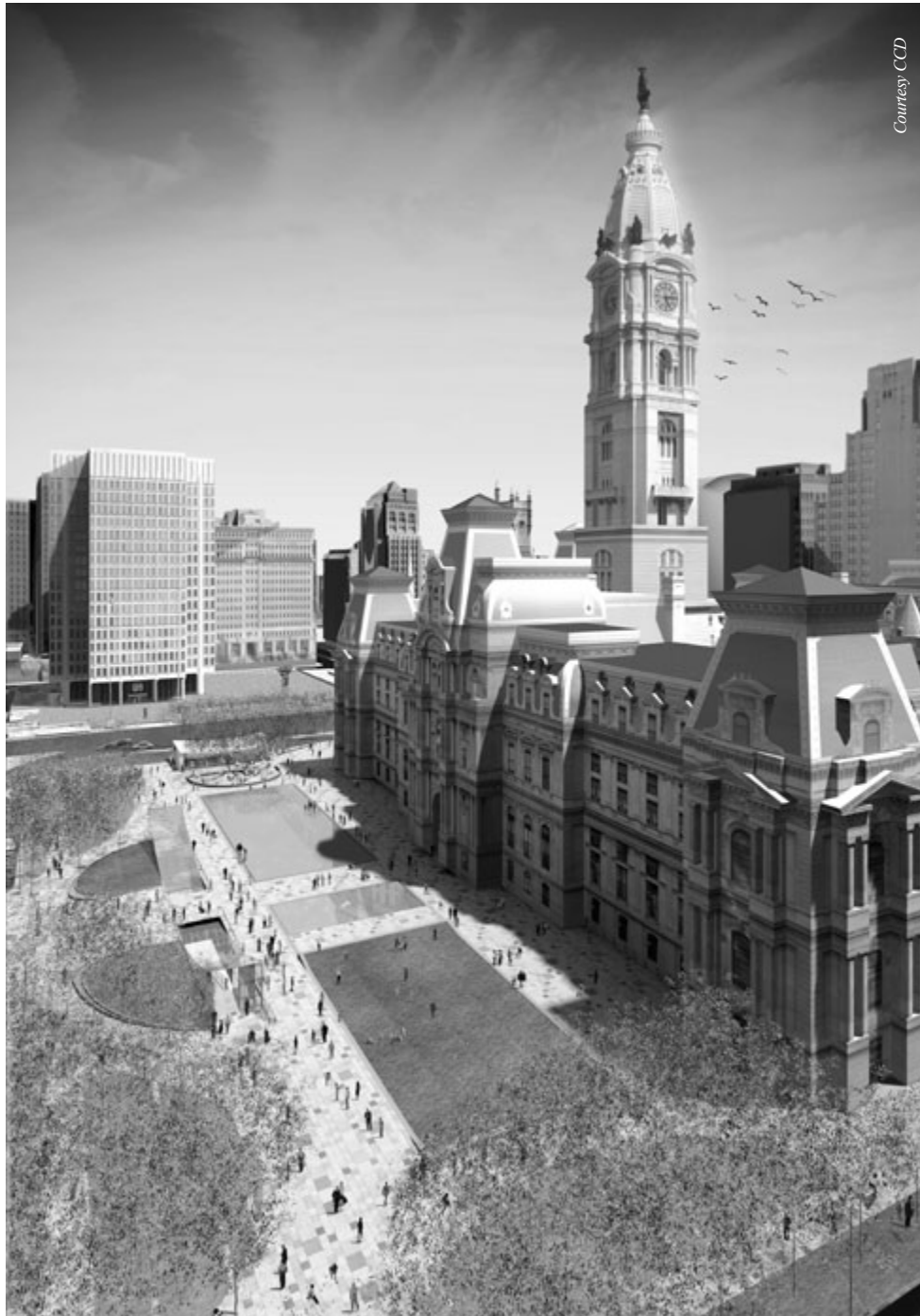
With a lawn at the south end and a café and programmable fountain at the north, Dilworth Plaza is planned as a quiet space that from time to time can accommodate events such as concerts and seasonal markets.
