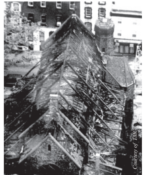
The morning after: charred beams are all that remain of the church roof.
