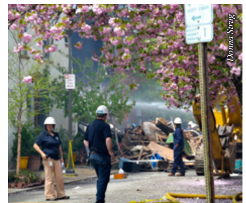
Utility workers observe the scene, while water is sprayed on the site of the explosion.
